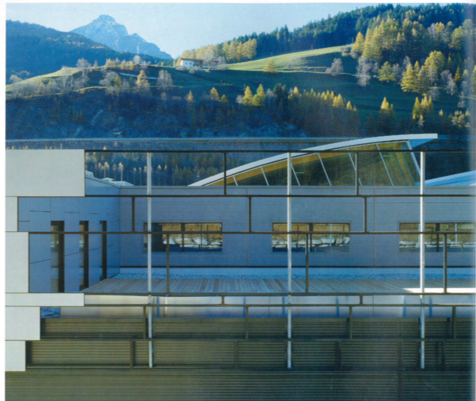
↑ | Shed roof of production hall → | Production hall with façade band
