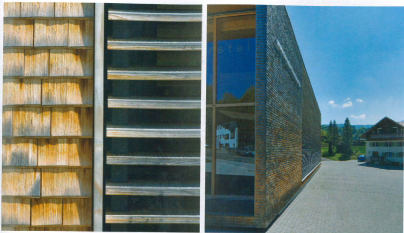
↑ | Detail of façade, timber fins and shingles
