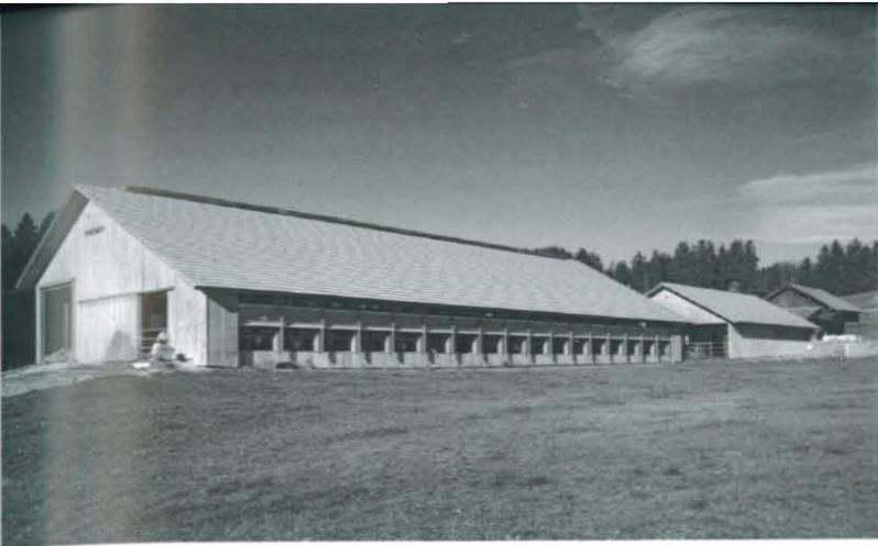
**Außenklimastall und Melkhaus in linearer Addition zu einer bestehenden Scheune am Rande einer Wiese | Naturally ventilated stall and milking house as linear addition to existing barn at the edge of a meadow**
